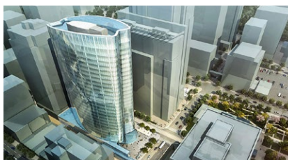
View of the 707 Fifth looking north west
