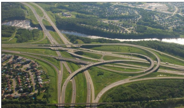
Fig. 5: The A20/A73 Highway Interchange in Levis, Quebec. Another structure seismic isolated with LRBs by mageba
